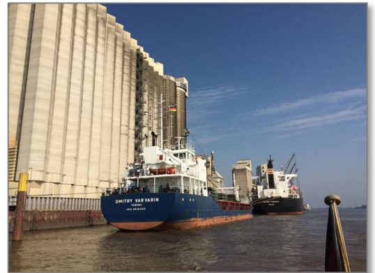
Providing robust RTK next to silos in Brake's pier
